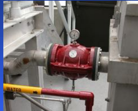
Pinch Valves: Forgiving, simple, and durable
