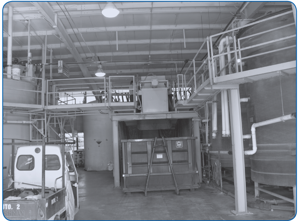
Inside a portion of the Kline Services facility.
