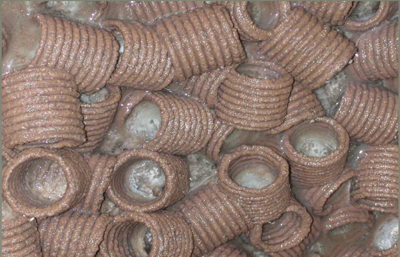
Surface of trickling filter organically overloaded
