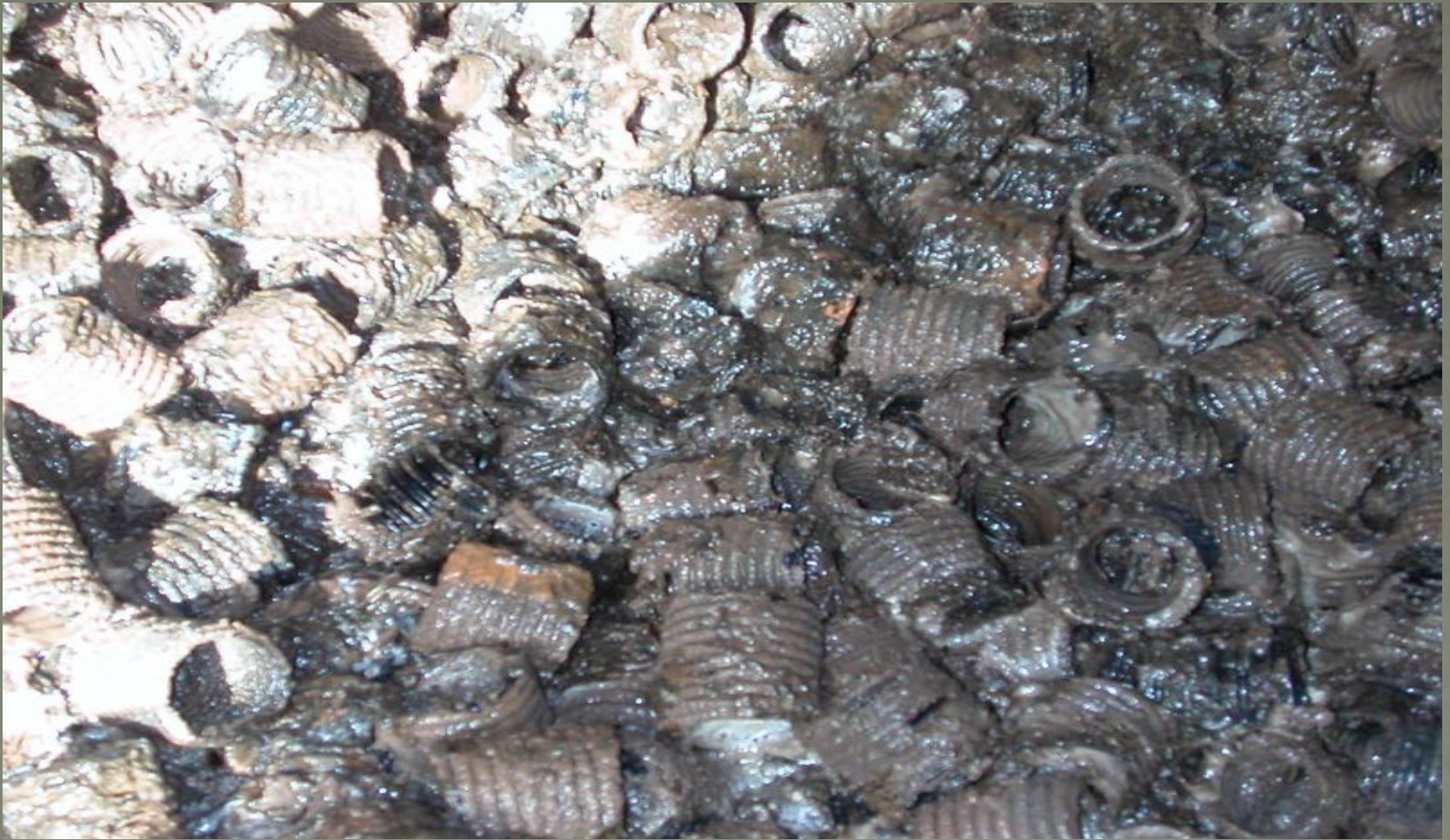
Organically overloaded trickling filter beneath the surface
