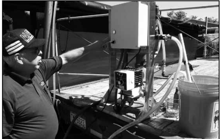
Get first-hand experience with septage and grease trap treatment during up-close demonstrations of equipment at a working facility.
